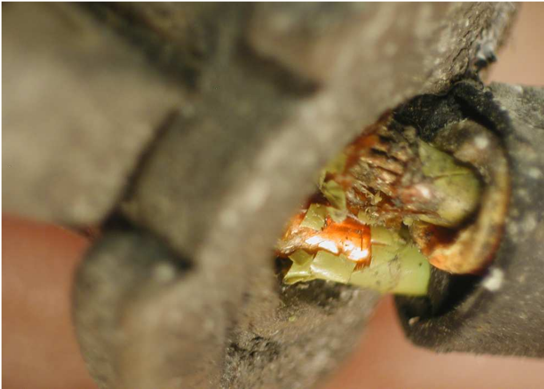
Figure C-9: Harness: H16DW693-21. Wires coming out of a conduit with multiple breaches to conductor.
