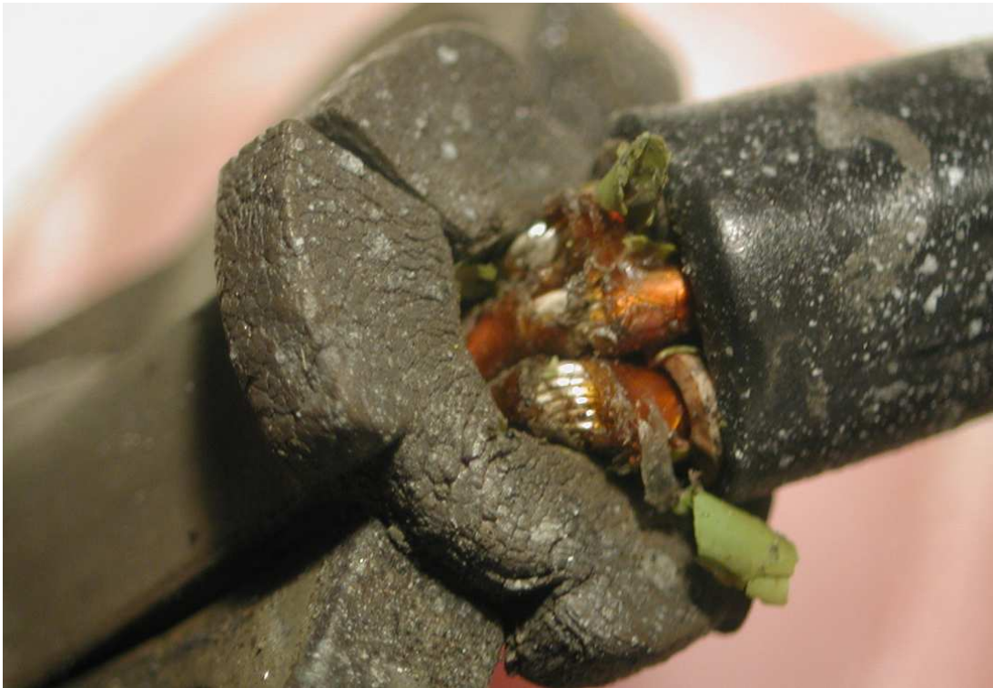
Figure C-10: Harness: H16DW693-21. Same as Figure C-9.
