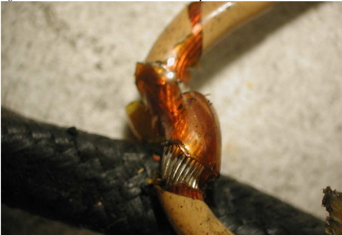
Figure C-2: Photo: Harness: H16DW685-23: Photo taken under higher magnification. Conductor exposed.
